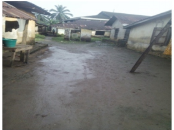
Plate 3: Abandoned Buildings in Nkemba Lane
